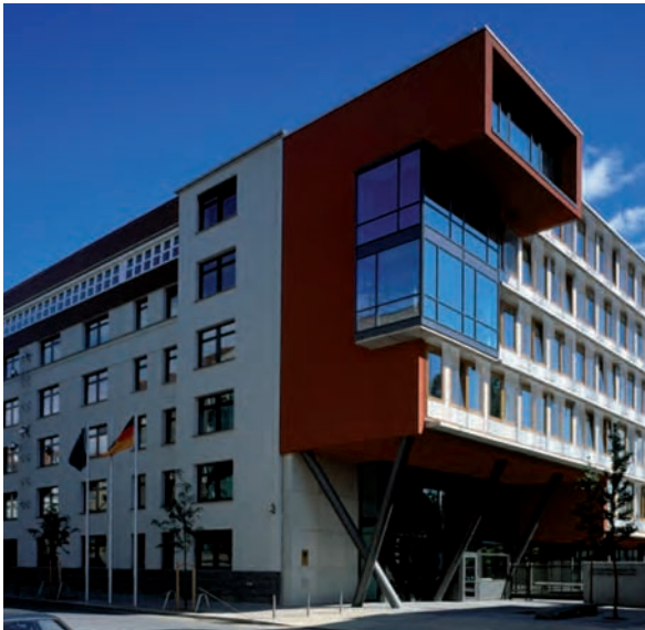
The BMBF building in the Hannoverschen Strasse 28-30, Berlin
