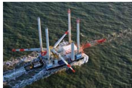
Germany's first offshore wind power plant.
